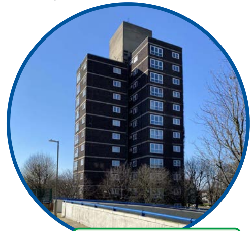
Tall buildings are a feature on the estate
